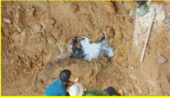
The underground gasoline tank at the petrol station broke due to severe rust on the tank wall. Underground water seriously polluted in the large area (Yen Bai province)
