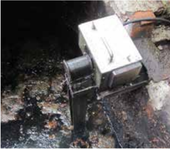
Oil skimmers installed in the oily wastewater collection tanks of mechanical repair workshops
