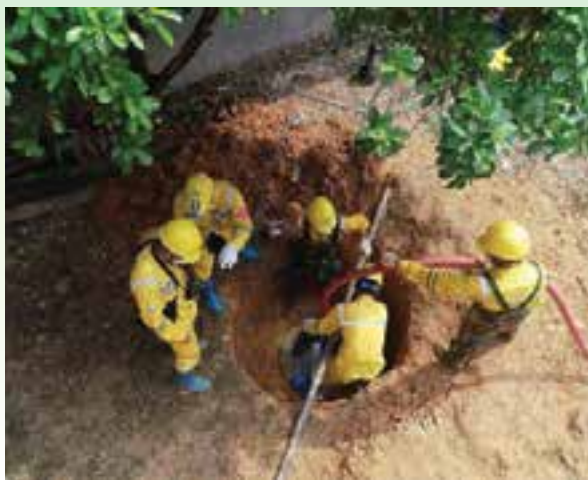
Use C-PEC to treat oil-contaminated groundwater
