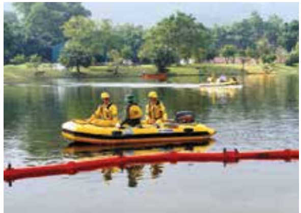
Deploy flat oil containment booms in oil spill emergency response on lake
