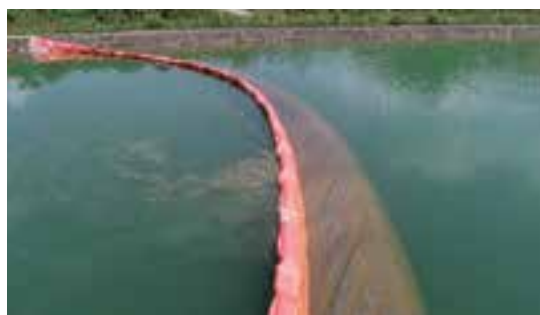
Oil filtering fabric combined with oil containment booms to proactively prevent oil pollution in the water intake canal of a water plant
