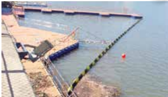
Permanent oil containment booms installed at the cooling water intake area of a thermal power plant
