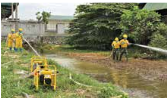
Use SOSE-7 to high-pressure wash oil-contaminated ditches
