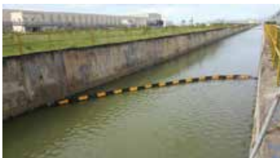
Permanent oil containment booms installed at the drainage canal of a petrochemical refinery
