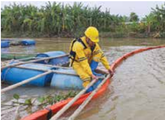
Use flat oil containment booms to isolate oil contaminated areas on river
