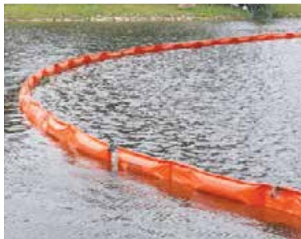
Deploy oil containment booms in oil spill emergency response on lake
