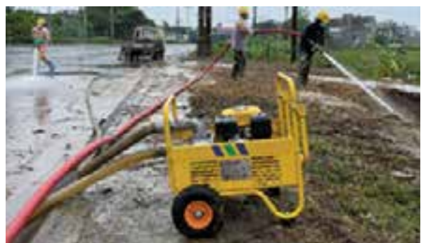
Use SOSE-7 to high-pressure wash oil-contaminated ditches and roads
