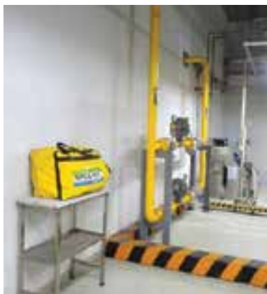
Spill kits equipped at chemical spill risk points of medical equipment factory
