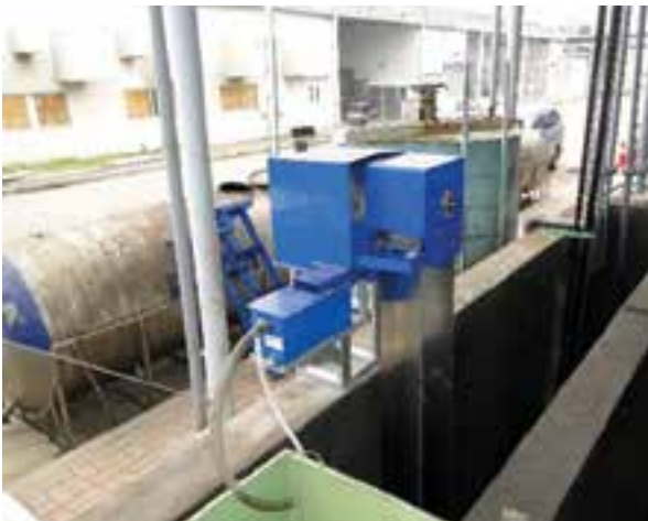
Oil skimmers installed in the oily wastewater collection tanks of mechanical repair workshops
