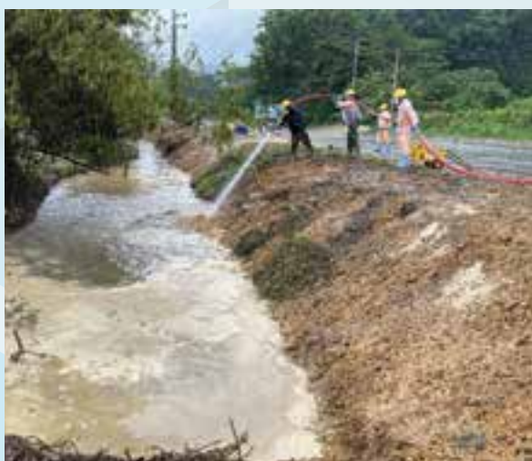
Spray HAZO to eliminate gasoline vapor dispersion and prevent the risk of fire and explosion during oil spill emergency response
