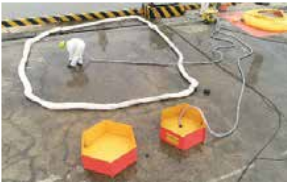
Deploy hexagonal tanks to store oil collected from oil spill response activities at port
