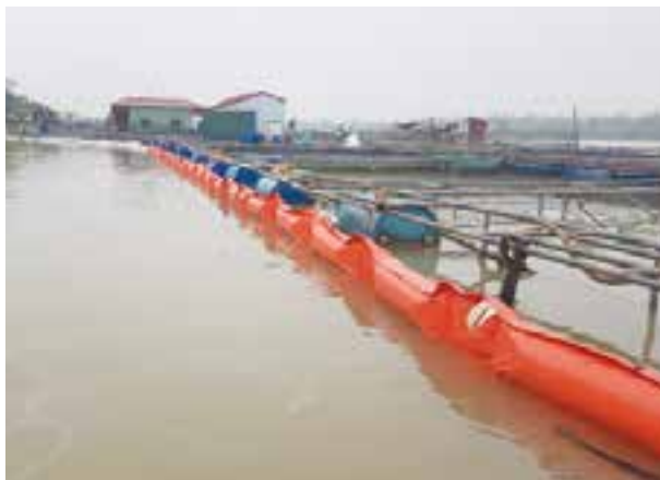
Deploy oil containment booms to protect fish cage areas from being contaminated with oil scum
