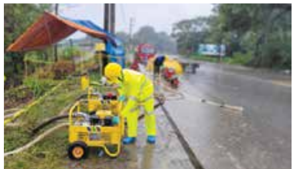
Use SOSE-2 to recover spilled oil at irrigation ditches
