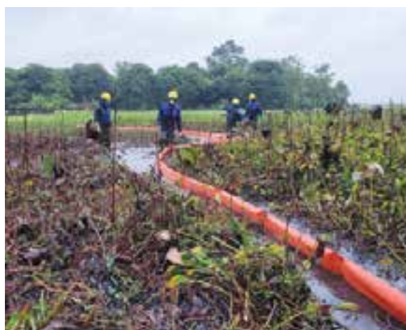
Use flat oil containment booms to isolate oil contaminated areas on agricultural land
