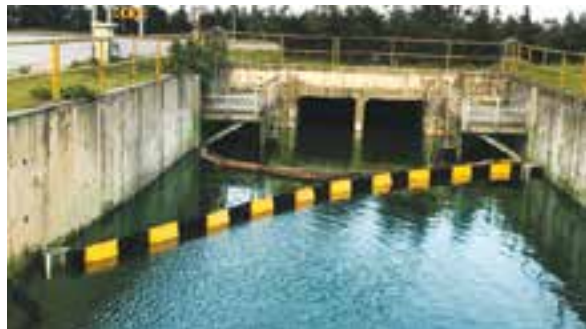
Permanent oil containment booms installed at the drainage canal of a steel factory
