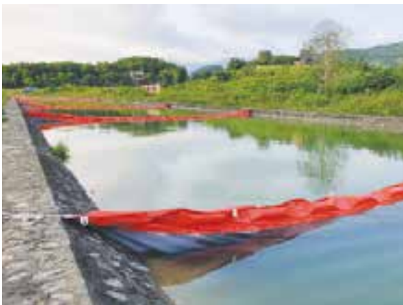
Use oil containment booms combined with oil filtering curtains to proactively prevent oil pollution in the water intake canal of a water plant
