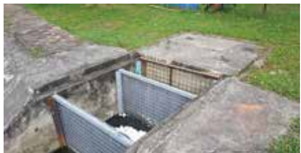
Oil filtering frames at an industrial park's discharge sewer
