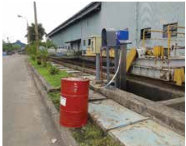
Oil skimmers installed in the oily wastewater collection tanks of mechanical repair workshops
