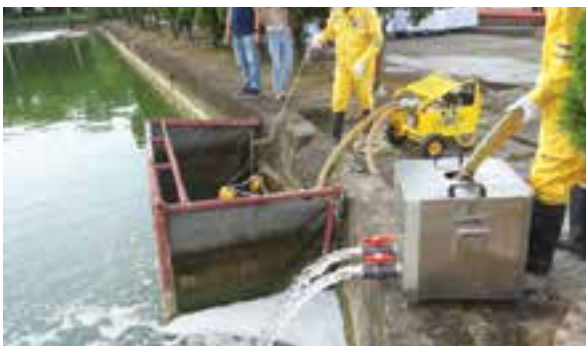
Use SOSE-2 to recover spilled oil at the stormwater collection gate of a petroleum depot
