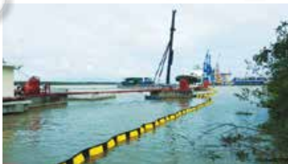
Permanent oil containment booms installed at an aviation fuel port
