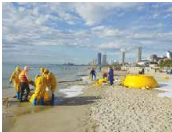
Use mobile tanks to temporarily store oil-contaminated water recovered from oil spill response activities at the coastal area
