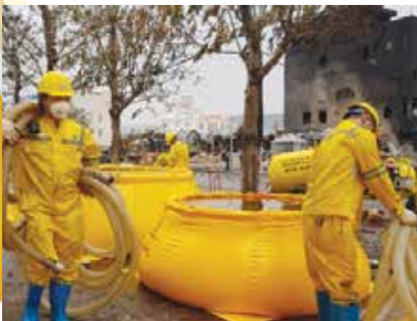
Use mobile tanks to temporarily store oil-contaminated water collected from oil recovery activities after a fire incident
