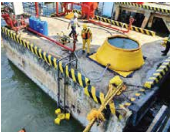
Deploy mobile tank to store oil recovered from oil skimmer at a port
