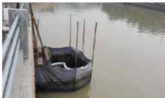
Oil filtering layer at the discharge drain of a thermal power plant
