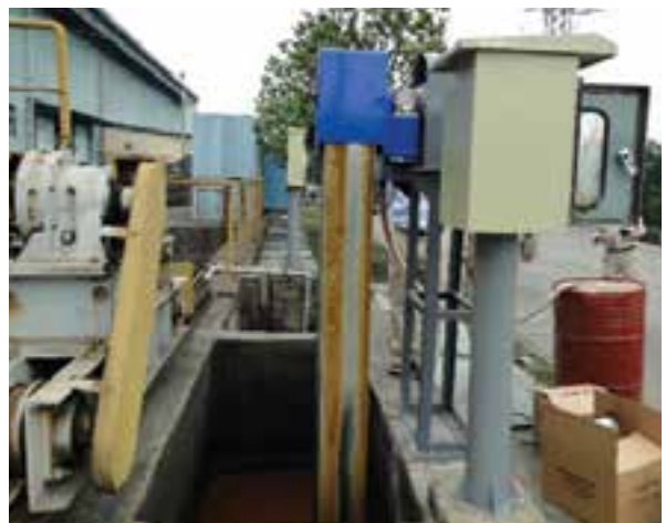
Oil skimmers installed in the oily wastewater collection tanks of mechanical manufacturing factories
