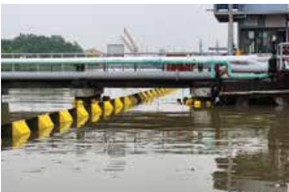
Permanent oil containment booms installed at a petroleum port
