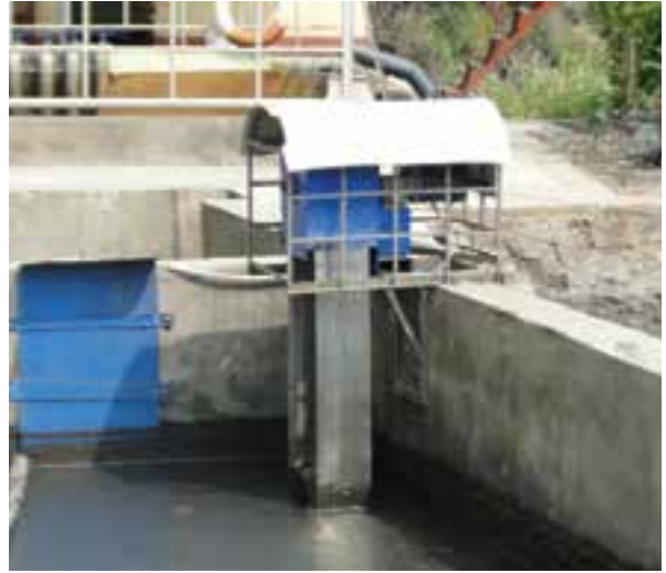
Oil skimmers installed in the oily wastewater collection tanks of mechanical repair workshops
