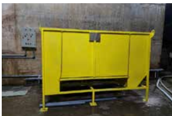
Using oil-contaminated wastewater treatment module for on-site treatment of oil-contaminated water at hydropower plants
