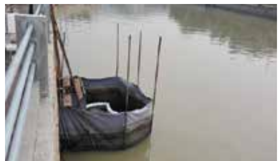
Oil filtering layer at the discharge drain of a thermal power plant
